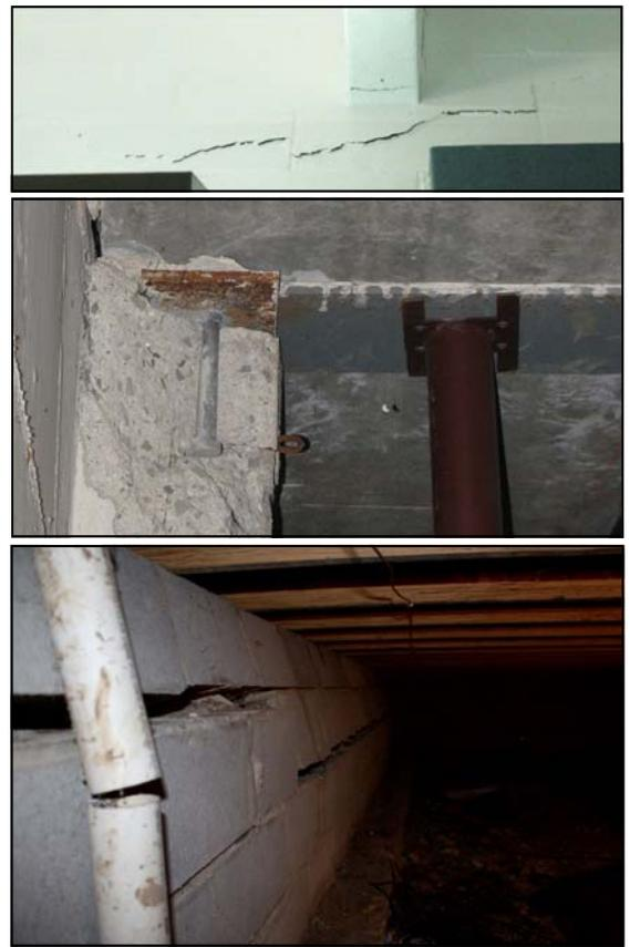
FIGURE 3 EXAMPLES OF STRUCTURAL DAMAGE
