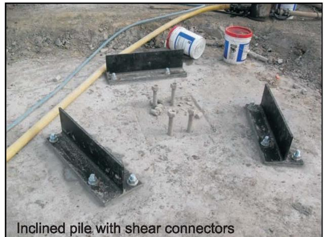
FIGURE 3: FOOTING SUPPORTED ON THREE PILES
