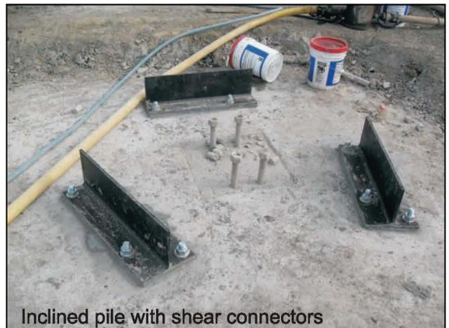
FIGURE 3: FOOTING SUPPORTED ON THREE PILES
