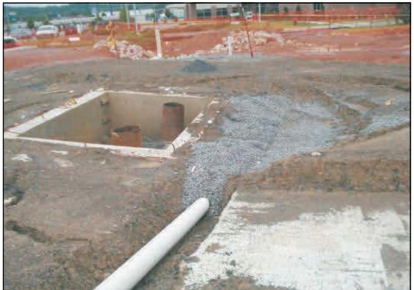
FIGURE 1: PICTURE SHOWING SAG SUBSIDENCE WHICH FORMED DURING CONSTRUCTION AND ENCOMPASSED AN ELEVATOR PIT
