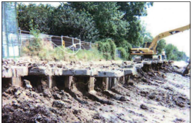
FIGURE 5: EQUIPMENT SUPPORT MOVED DOWNWARD AND OUTWARD DURING DRY SLOPE CONSTRUCTION
