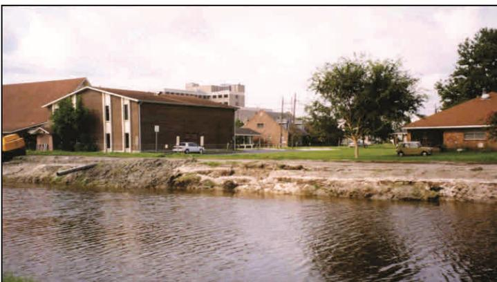
FIGURE 3: FAILED CANAL BANK DURING CANAL BOTTOM CONSTRUCTION
