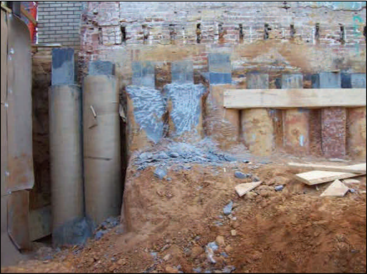
FIGURE 3: SUCCESSFULLY INSTALLED MODIFIED SECANT WALL CONSISTING OF STIFF CONCRETE SHAFTS THAT PROTECTED IMMEDIATE EXISTING BUILDINGS
