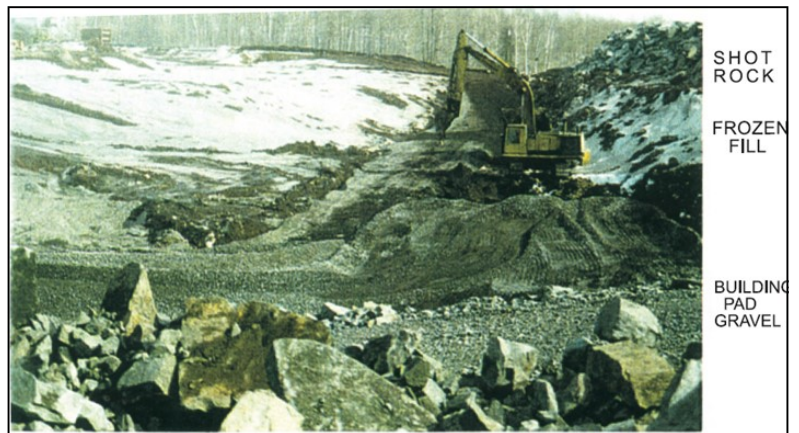
FIGURE 6 GRAVEL BEING INSTALLED IN BUILDING PAD AND AGAINST FROZEN FILL SLOPE
