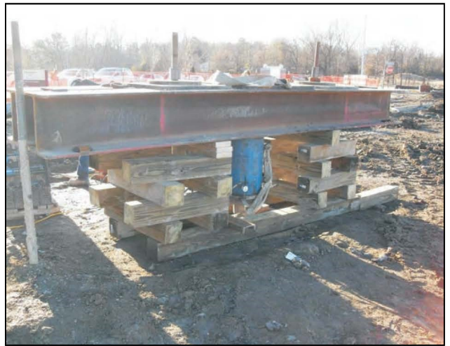
FIGURE 2: PILE VERIFICATION TEST SETUP
