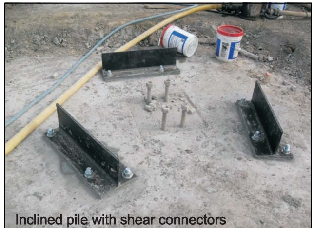
FIGURE 3: FOOTING SUPPORTED ON THREE PILES
