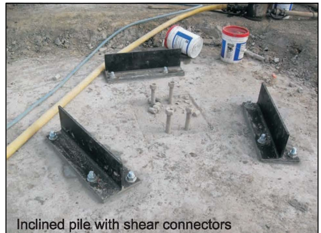
FIGURE 3: FOOTING SUPPORTED ON THREE PILES
