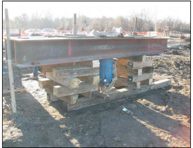
FIGURE 2: PILE VERIFICATION TEST SETUP
