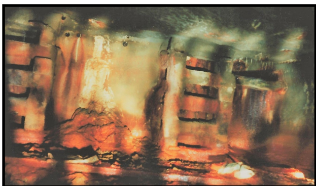
FIGURE 3 DOWNSTREAM SEEPAGE EFFECTS AT SEAL NO. 7. PHOTO TAKEN AFTER FAILURE
