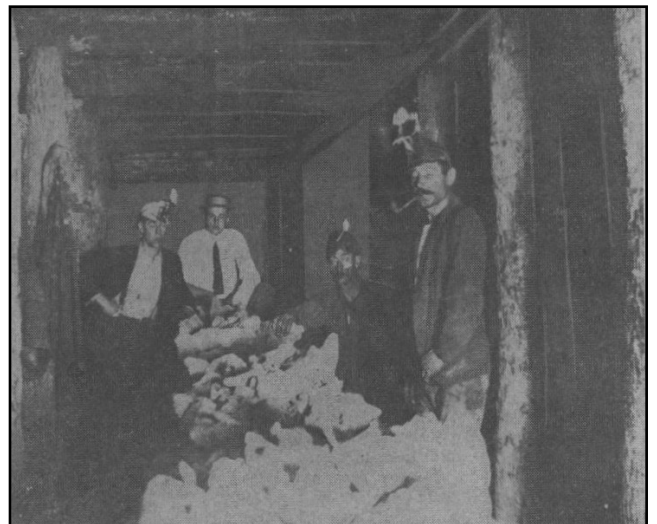
FIGURE 1 WORKERS STANDING ALONGSIDE CLAY CARTS IN ONE OF THE HIGHLANDS FIRECLAY COMPANY'S TUNNELS UNDER THE OLD FOREST PARK HIGHLANDS IN 1908. Photo by Sam Leone. From: https://bit.ly/2Wwn4ZA
