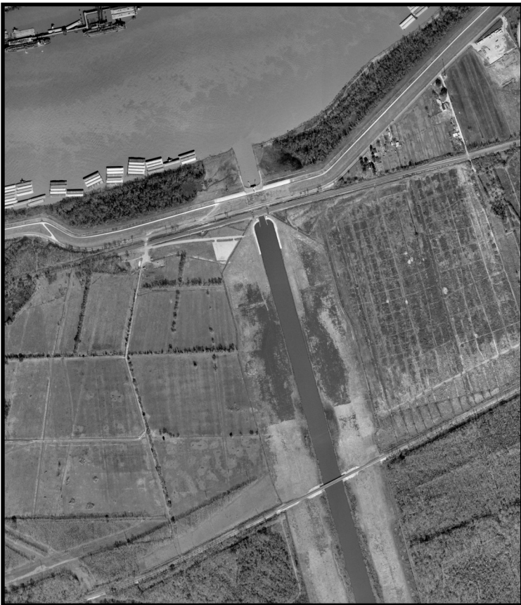
FIGURE 2 AERIAL IMAGE OF CONSTRUCTION OF THE DIVERSION STRUCTURE COMPLETED
