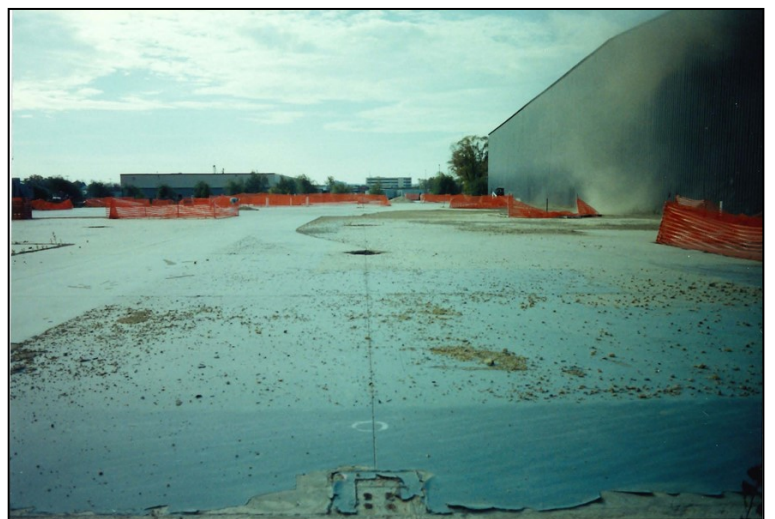
FIGURE 5 SOUTH VIEW OF DISMANTLED STRUCTURE
