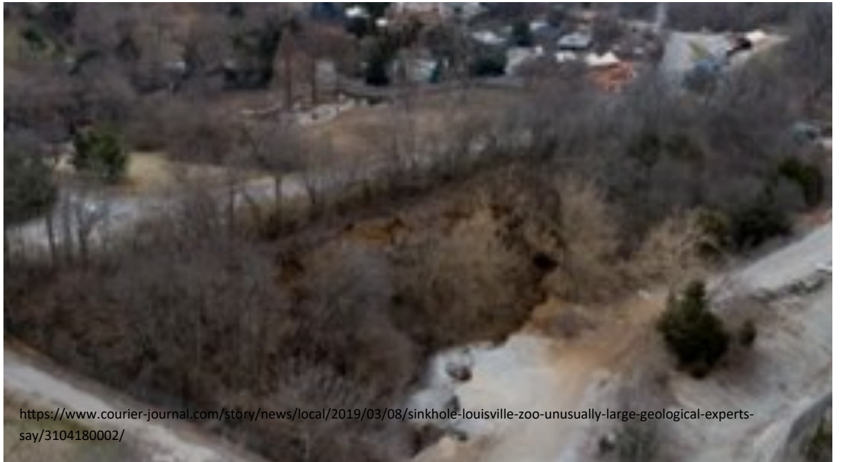
FIGURE 1 40FT CRATER WHICH FAILED OVER A LIMESTONE MINE
