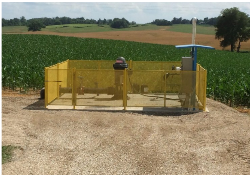
FIGURE 3 SURFACE DECANT HOLE SETUP
